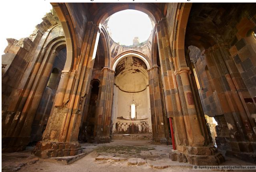
Fig. 10. Interior of Ani Cathedral (1001 AD). The pendentives on which the dome is rested are clearly visible. The clustered piers, the pointed arches and vaults remind one of early Gothic architecture but these forms appear in Armenia about 100 years before Western Europe (Author).
