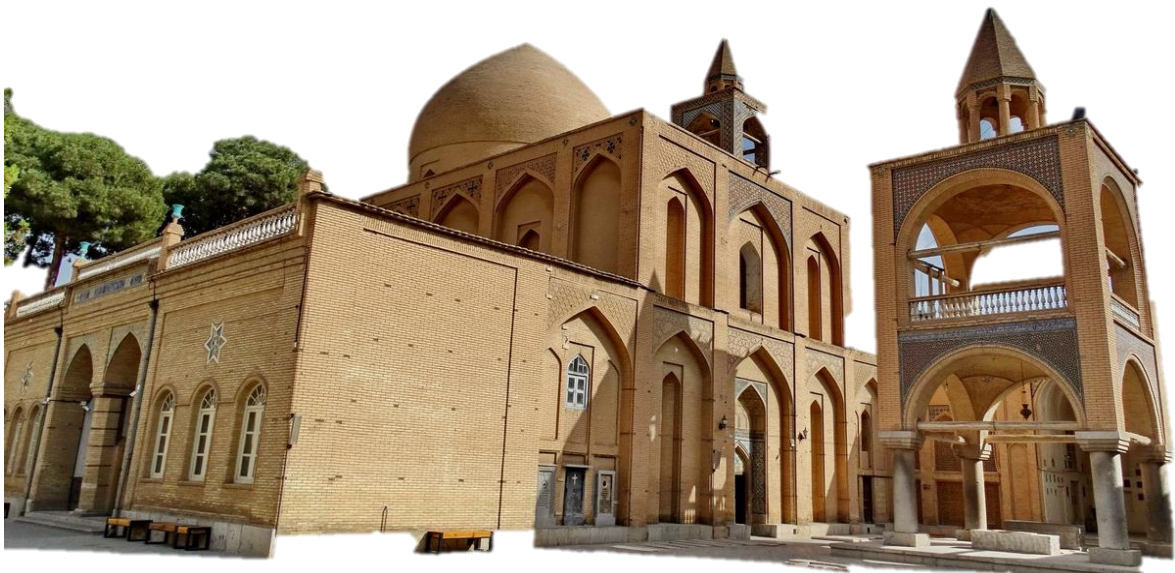
Fig 13. Vank Cathedral bell tower (1702), Armenian in form but Iranian in material (brick). Note the Safavid blind pointed arches on the left wall (Author 2008).
